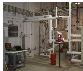
Absorption Cooling System
