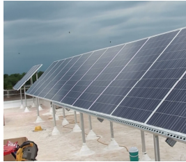
PV Solar Installation
