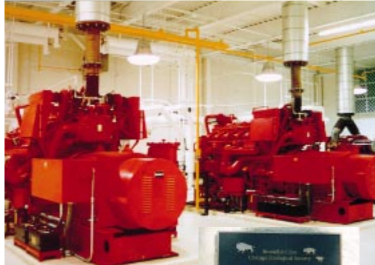
At the heart of the Brookfield Zoo's cogeneration plant are two Waukesha VHP7100GL Enginator® units.
